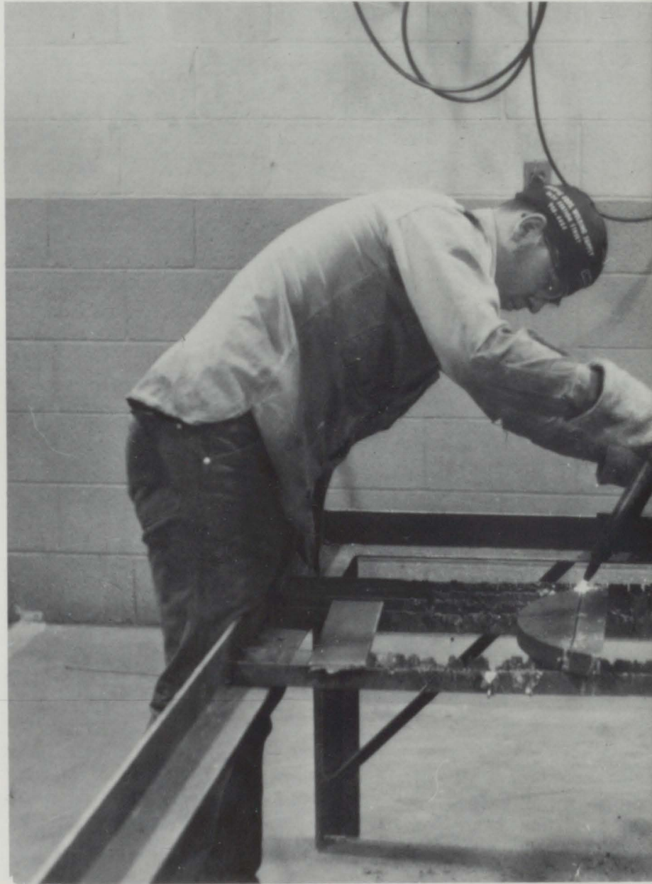
Top Right — Larry Hamilton is wearing a welder's mask to protect his eyes and face while welding.
